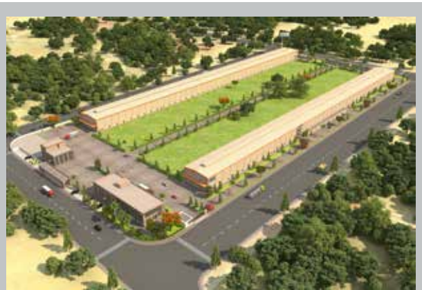
Jaipur Plant, India
