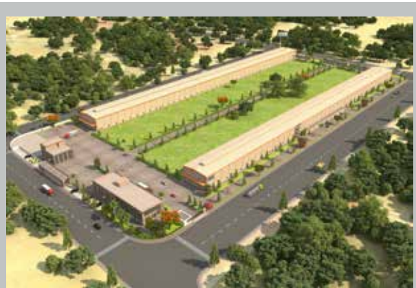
Jaipur Plant, India
